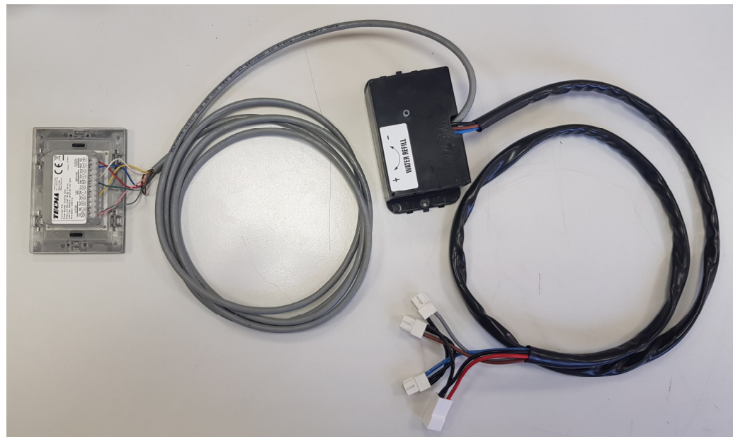
Previous Electrical Connections
